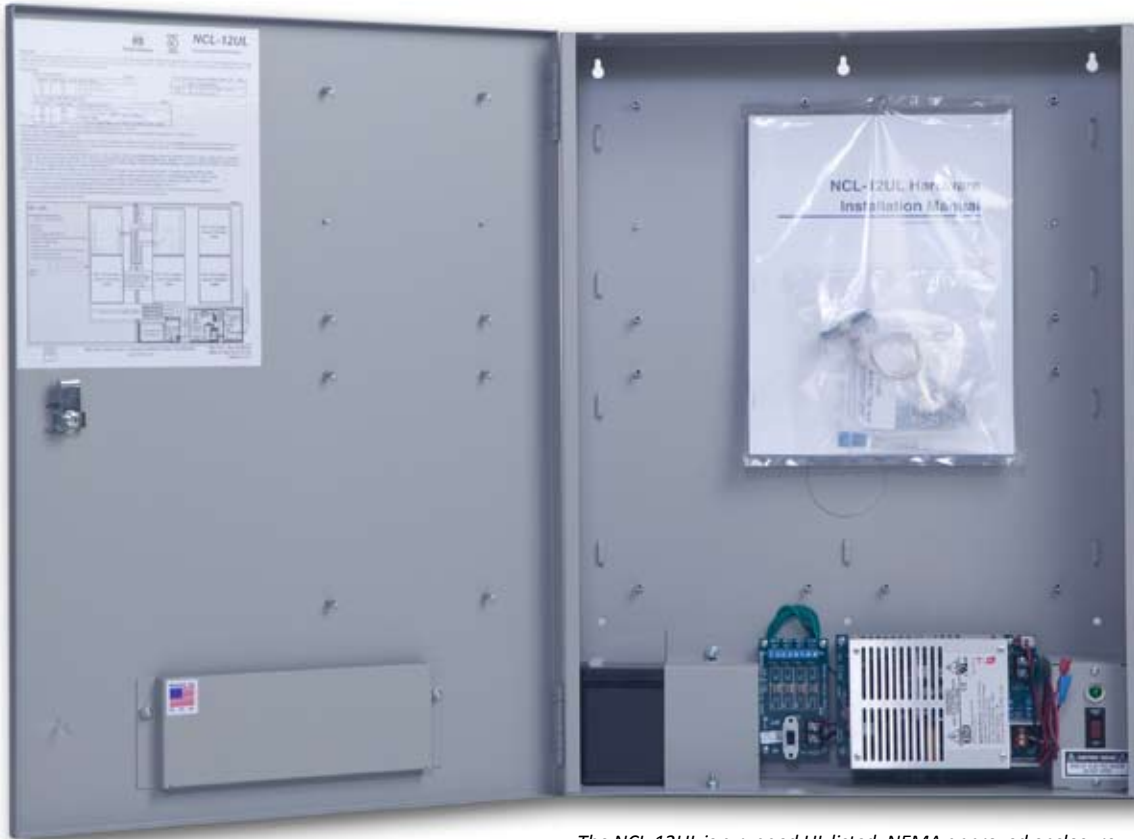
The NCL-12UL is a rugged UL listed, NEMA approved enclosure designed to accommodate up to six boards.
